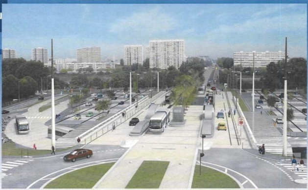
Nantes – the busway with articulated buses, implemented like the other tram lines, that will be opened the 6 th of November – 7 M€ / km
